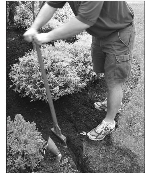
Pushing the tool back and forth widens the trench and creates a channel for the wire.
