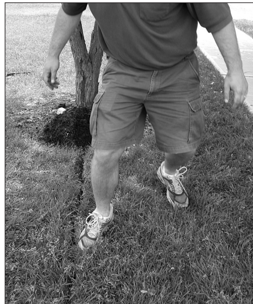
In turf, the trench is easily closed by gently pushing in from both sides.
