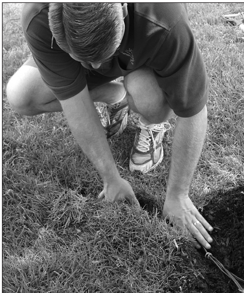
Wires are pushed firmly into the trench.
