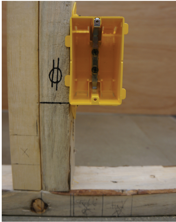
Figure 10 —Placement of box in relation to mark on stud
