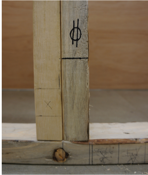
Figure 7—6" (15 cm) mark and a receptacle symbol
